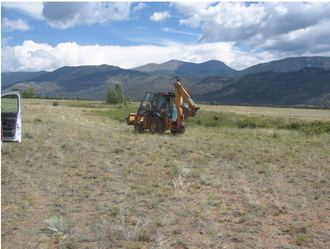
Soil Being Deployed Along the Reach
