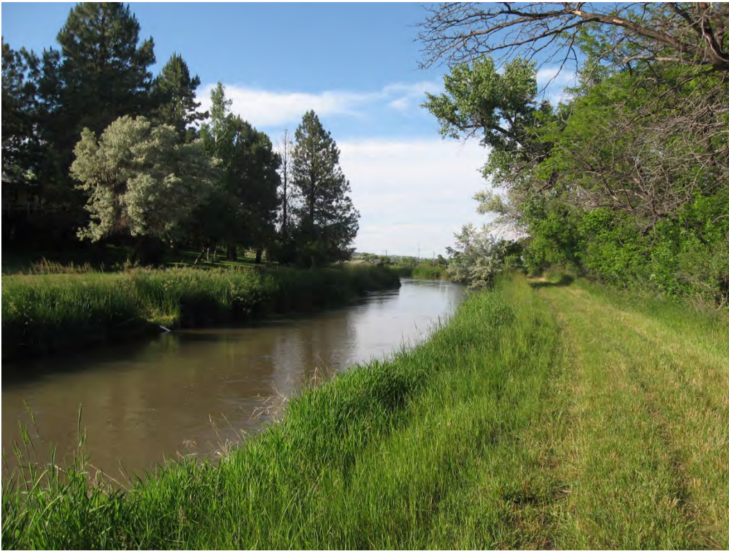
Upper Reach of the Canal before Application
