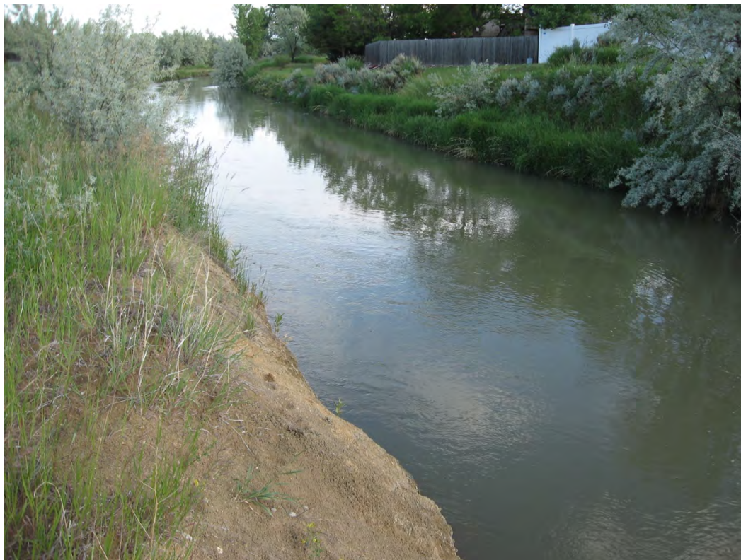
Lower Reach of the Canal after Application
